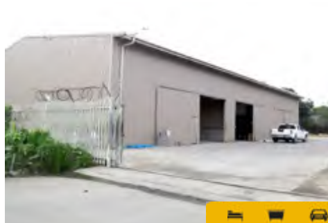
NM1356 - Warehouse in prime location - FN
