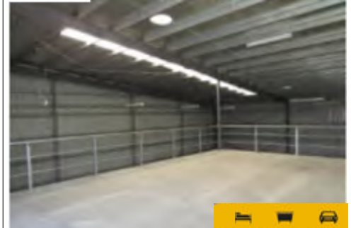
NM2080 - Warehouse close to the airport
