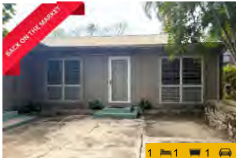
NM137 - Self-contained units - JTJ
